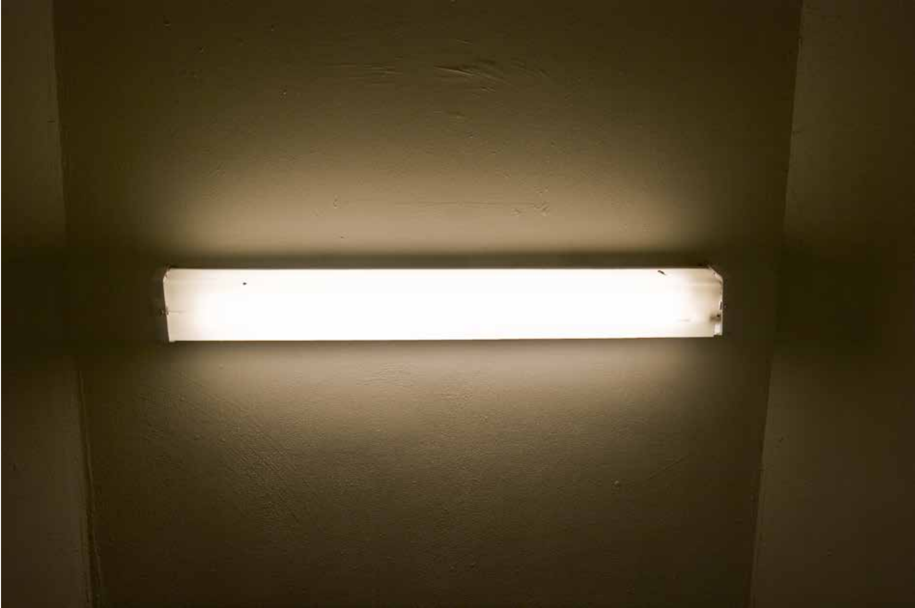
Stairwell Light, Center City Philadelphia
