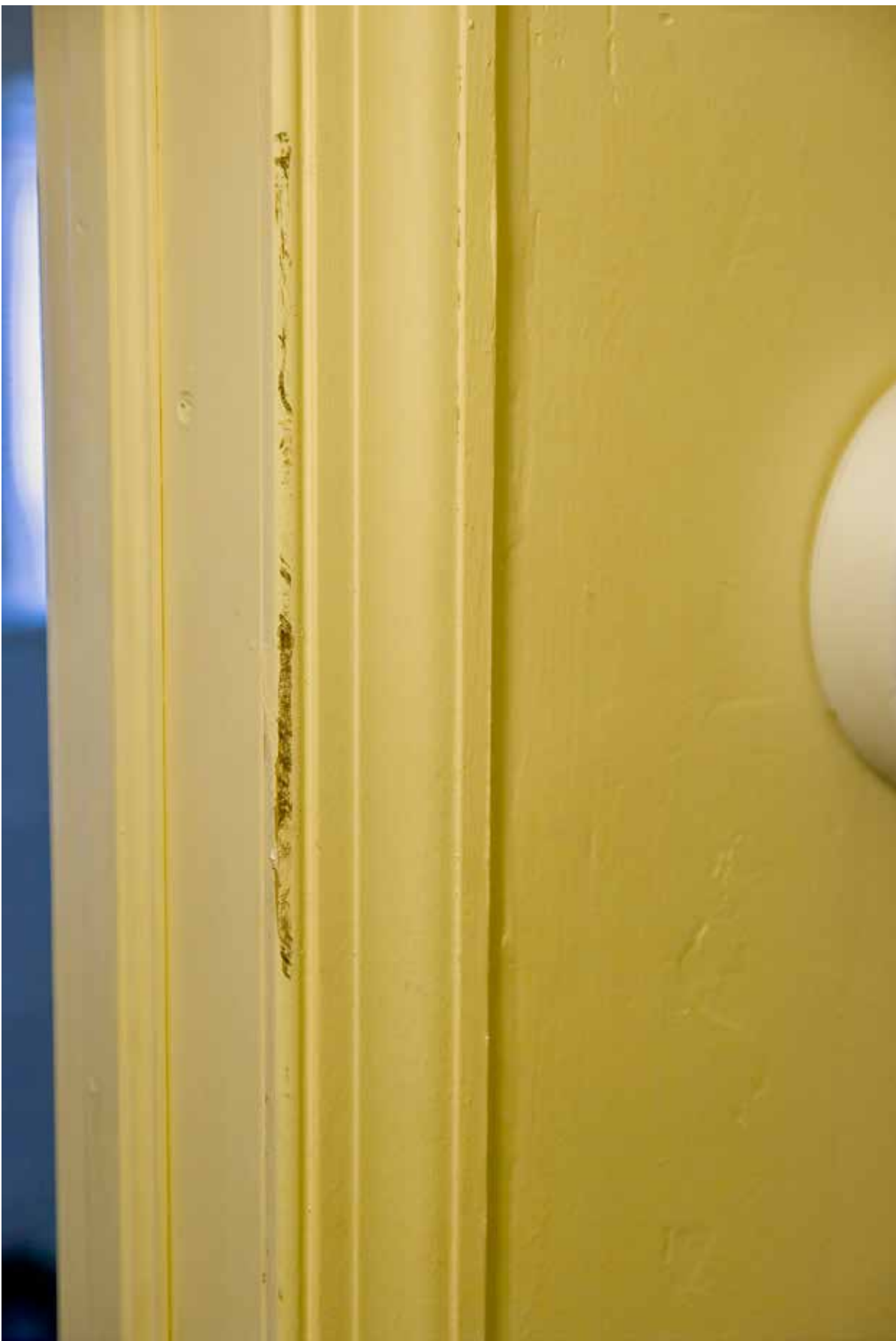
Damage, Fishtown, Philadelphia
